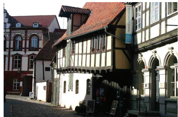
Time and gravity have yet to overcome these long-enduring structures.
